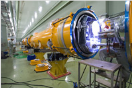
Crew welding the pipes at the far upstream end of the cryostat (TESLA-type cavity part).
