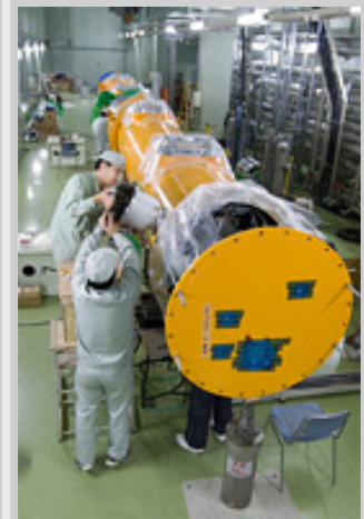
Crew installing the flange for signal cables on the cryostat (ICHIRO cavity part).
