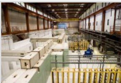
Getting ready to house the first cryomodules: Fermilab's ILCTA.
