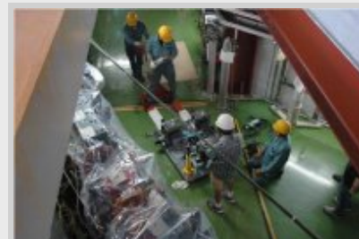
Installing the first test cavity in the ATF damping ring
