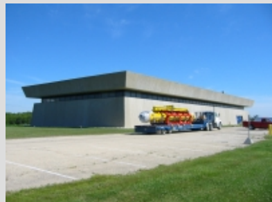
The first cryomodule on its way into the NML hall at Fermilab... (Photo: Fermilab)
