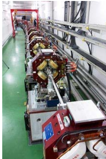
The Accelerator Test Facility 2 in Japan uses a 50-meter series of magnets to focus its electron beam. (Photo by N. Toge, KEK. Click for larger image.)
