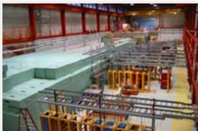
The New Muon Lab is being developed at Fermilab; it is where we plan important SCRF systems tests in the period beyond 2012
